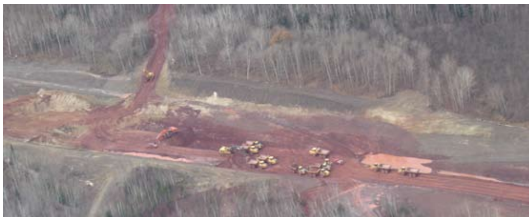
Excavators, trucks and dozers moved three million yards of soil along the 5.7 mile rail spur.
