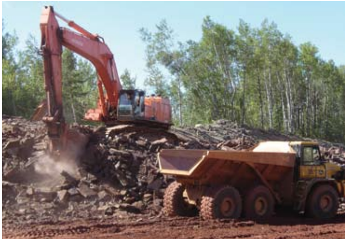
A Hitachi excavator loads one of our John Deere 400D ADTs.
