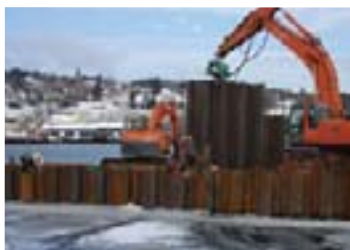
Sheet pile installation during winter...
